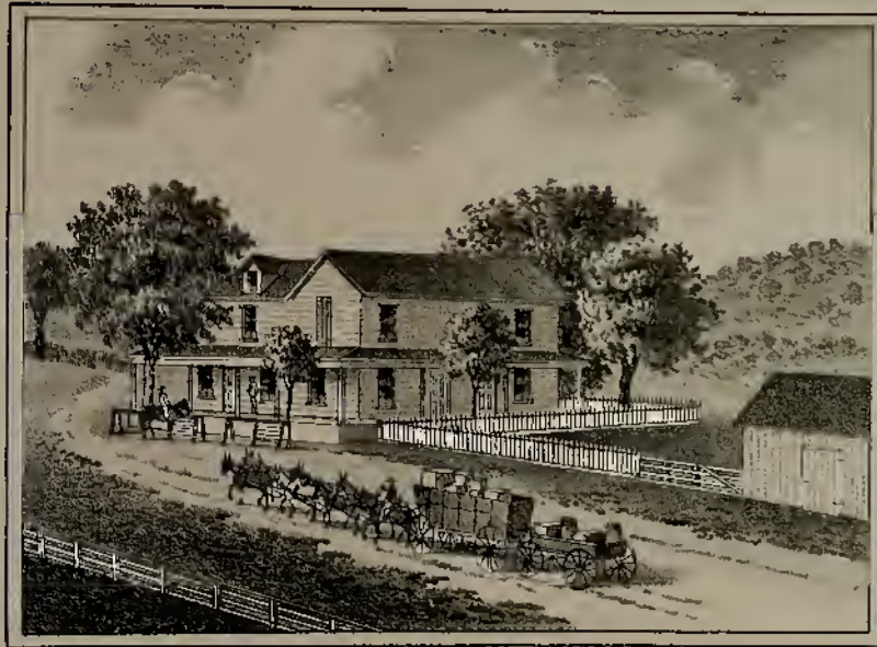
RESIDENCE OF W. T. FOSTER , CABBAGE PATCH, YUBA CO., CAL.
