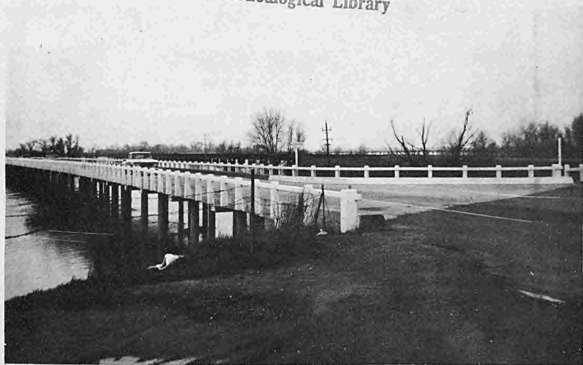
Long Bridge across By-Pass looking westward. Hwy. 20
