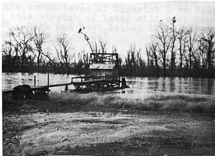
Sacramento River with a pump-house in foreground. At Tisdale Weir.
