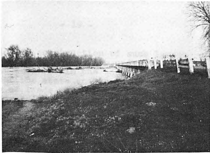
Water and debris going over Weir at Tisdale Weir. Water from river is entering the By-Pass.
