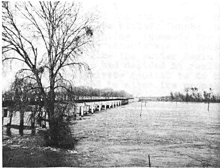
River water flowing into By-Pass at Tisdale Weir January 10, 1965
