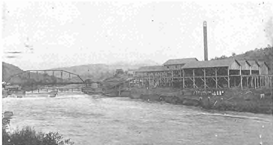
Klamathon Mill prior to 1900, showing County bridge and dam. (Courtesy Siskiyou County Museum)
