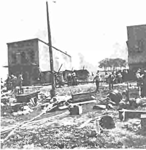
Waldon Bros. Store on left, remains of butcher shop in center and drug store on right. The fire was stopped at Waldon Bros. store.
