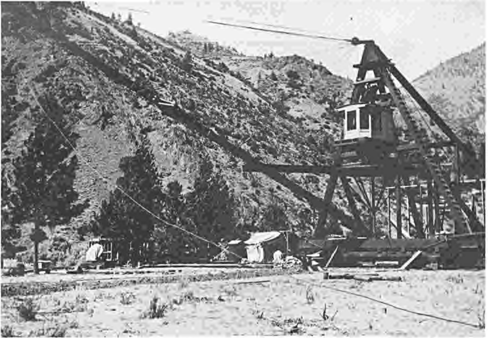
McConnell Bar Dredge. This was the first dragline to be used on the Klamath River. The dredge was invented and run by S.T. Wellman of Ohio for two and a half years below Humbug Creek. (Courtesy Chester Barton)
