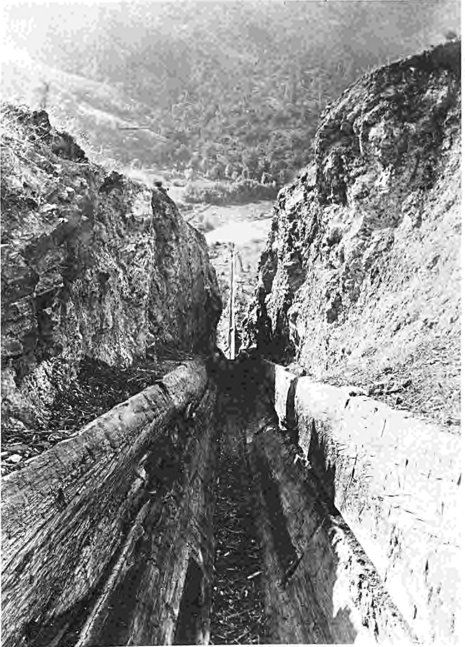
Top of log chute near Shovel Creek on Klamath River. From the top it was 2,650 feet to the river, with a vertical drop of 835 feet.
