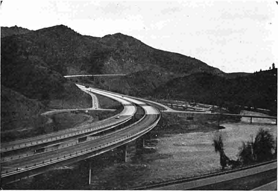
NOW: Interstate 5 bridges over Klamath River and Collier Rest Area on right. (Courtesy Darlene Anderson)
