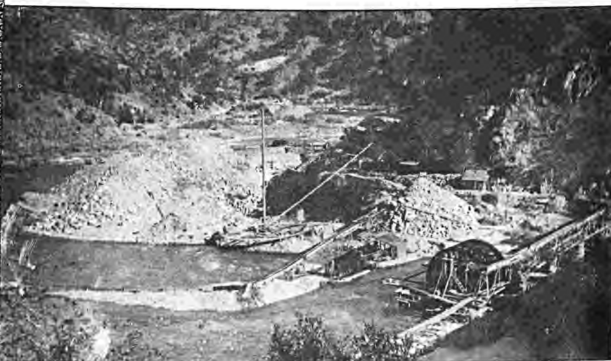
Power and dip wheel, showing how mining was accomplished on the— Klamath River.
