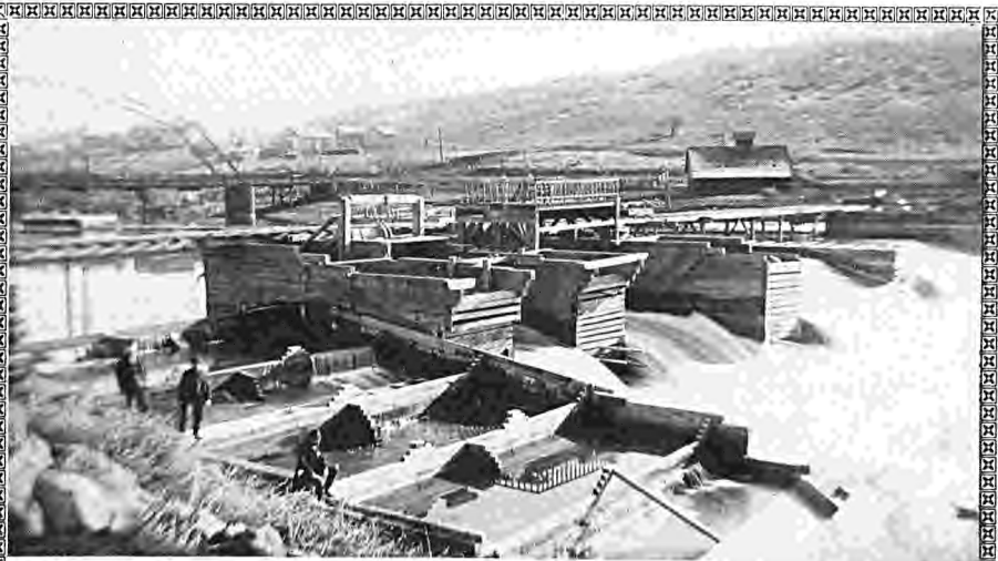
Klamathon, California, sawmill dam. Fish ladder to the left.
