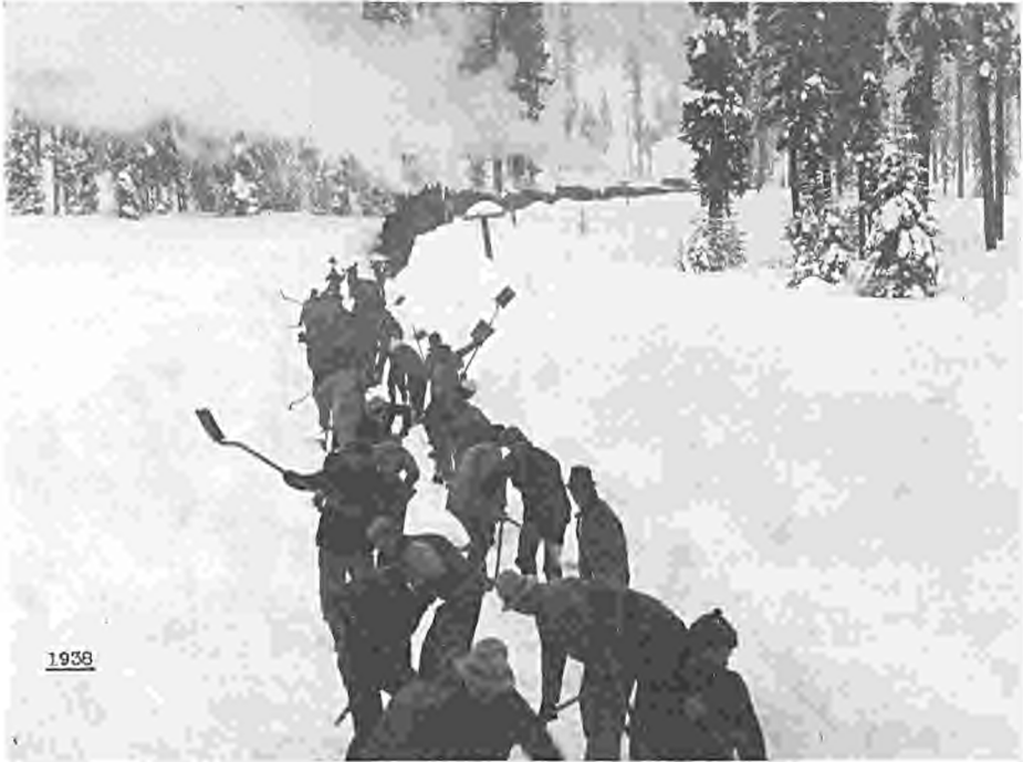
CLEARING THE TRACK FOR THE McCLOUD RIVER RAILROAD, 1938
