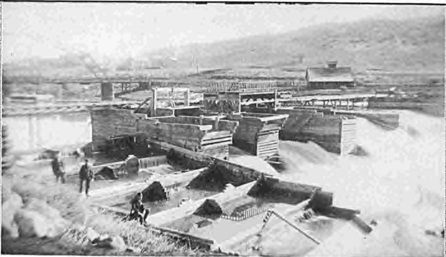
Klamathon Sawmill Dam. Note Fish Ladder on Left. —courtesy Siskiyou County Museum
