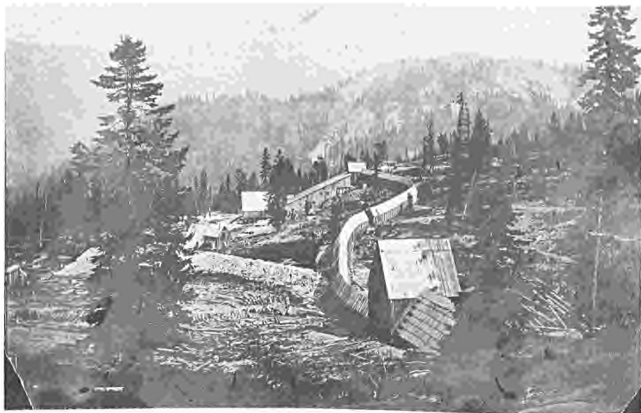
Dorleska Mill and snow shed. Covered track from mouth of tunnel to mill in background. —courtesy Mabel Frances Steele
