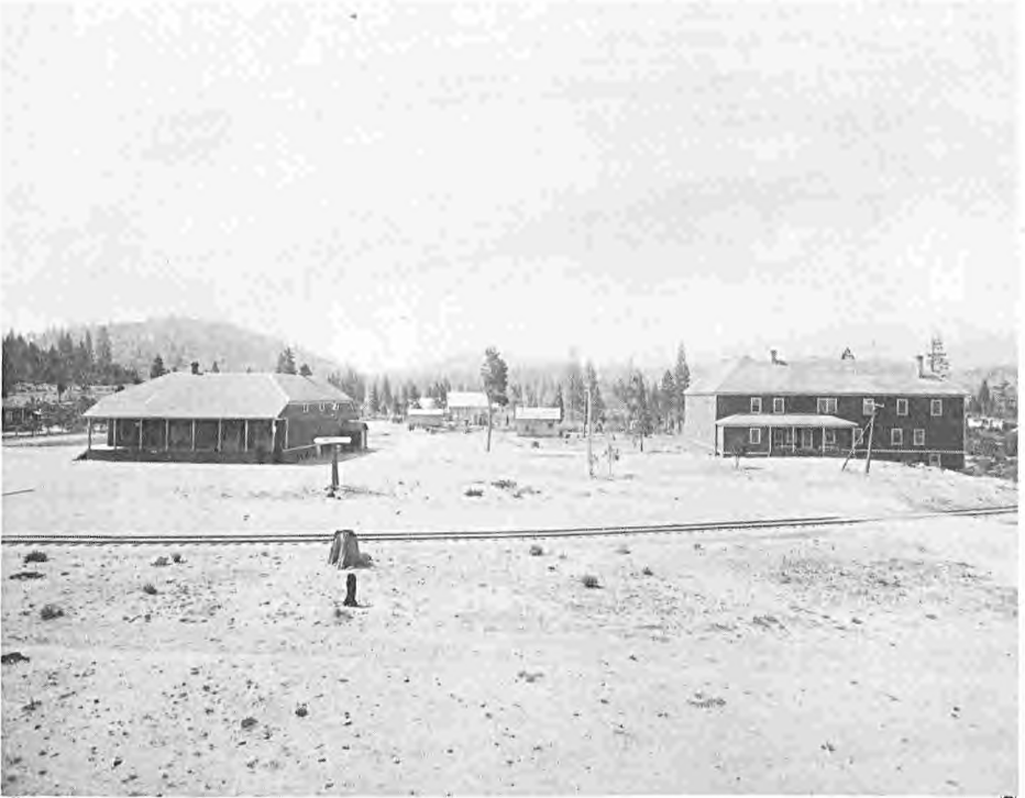
California Oregon Railroad in 1902. Road was completed through this area in 1887. Left is company store and post office. Right is factory boarding house operated by Paul and Phoebe Caulkett.
