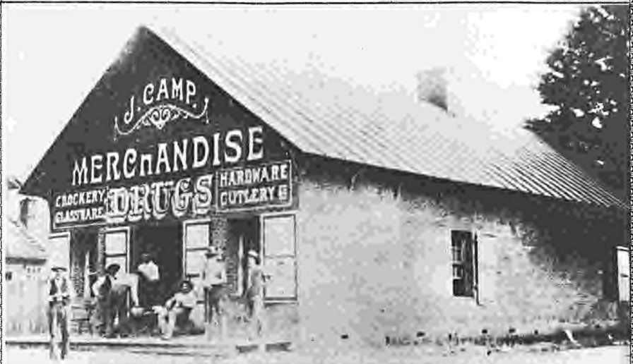
BRICK BUILDING BUILT IN 1862 AND STILL BEING USED.
