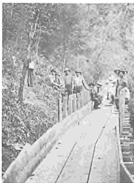
BUILDING THE FLUME FOR SISKIYOU MINES CO.
