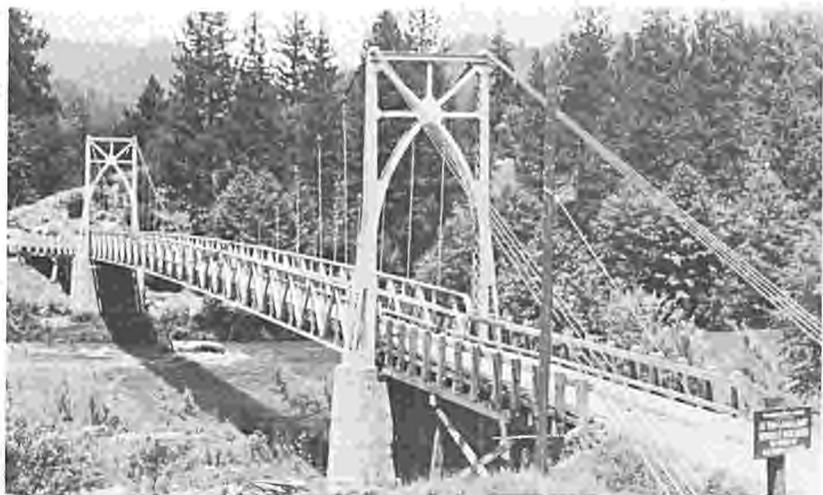
KLAMATH RIVER BRIDGE AT HAPPY CAMP
