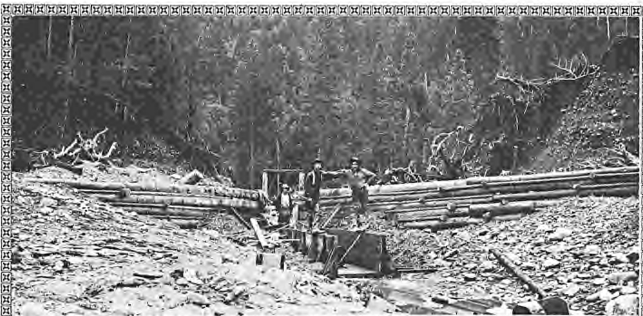
SETTING BOXES, SISKIYOU MINES, CLEAR CREEK
