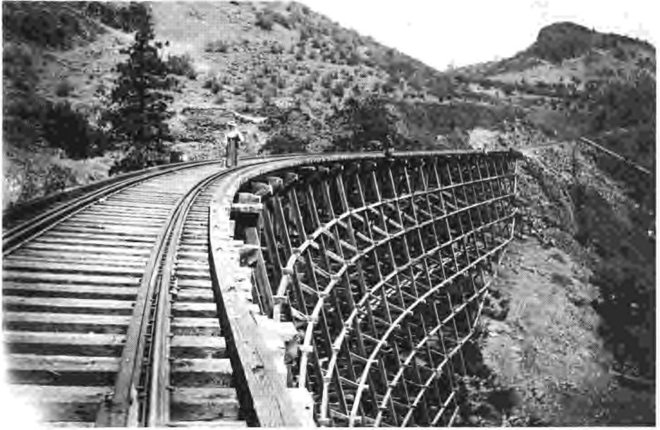
FALL CREEK TRESTLE
