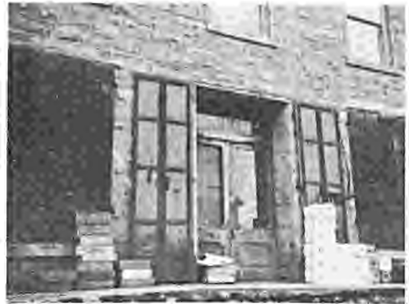
First Denny Bar Company store—iron doors were shutters for protection against the weather and, possibly, burglars.
