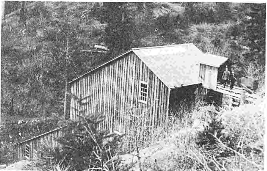
—courtesy Siskiyou Museum Dewey Mine—after cyanide plant was put in, recovered gold increased from $25 to $100 per ton.
