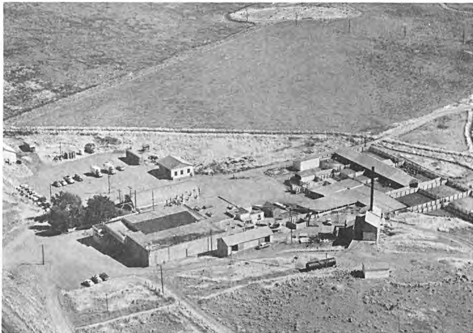
Aerial View of Plant.
