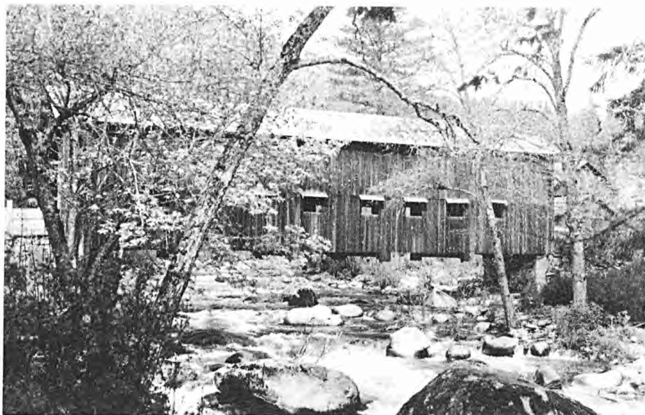
COVERED BRIDGE OVER THE LITTLE NORTH FORK OF THE SALMON RIVER.
