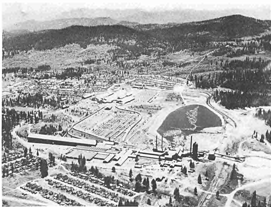
THE McCLOUD RIVER LUMBER COMPANY Aerial photo of the McCloud River Lumber Company mill and town.
