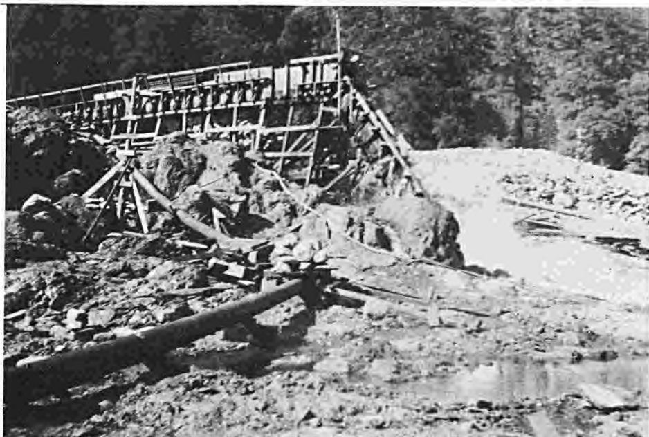
—courtesy Daggett Collection BONALLY PLACER MINE A hydraulic elevator at work at this North Fork mine in 1915.
