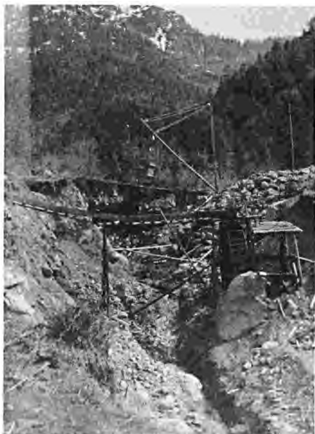
—courtesy Daggett Collection EDDY GULCH PLACER MINE The hoisting works in the foreground operated the crane in the background.
