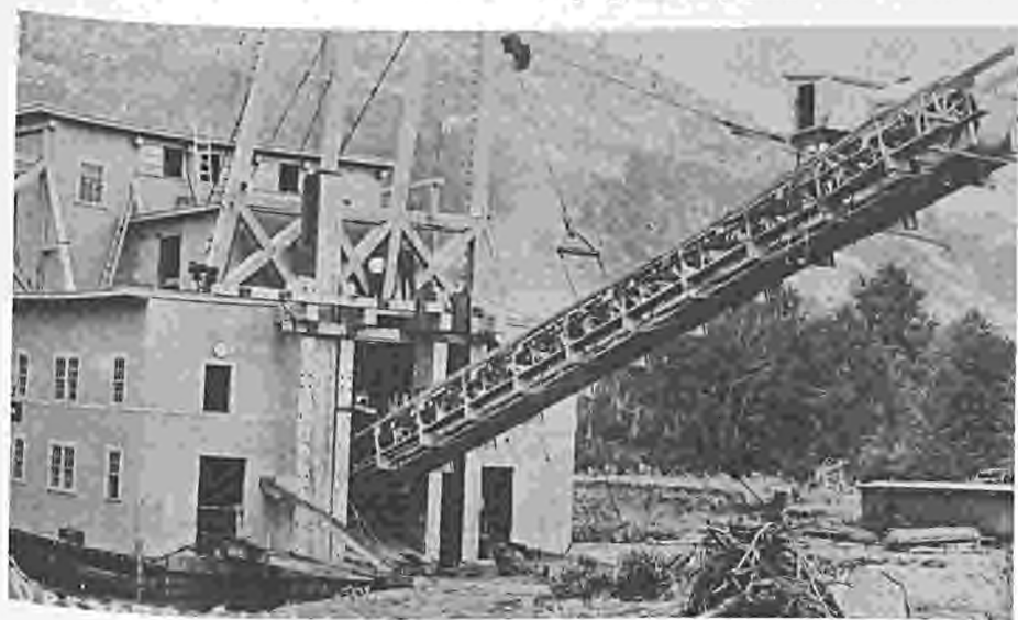
WADE DREDGE DURING CONSTRUCTION. Taken about 1907. Note 50-ton spud on right.
