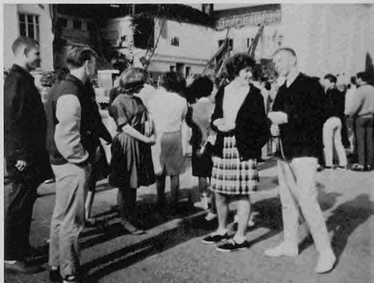
These Juniors don't appear too mournful about the demolition of old E.H.S.
