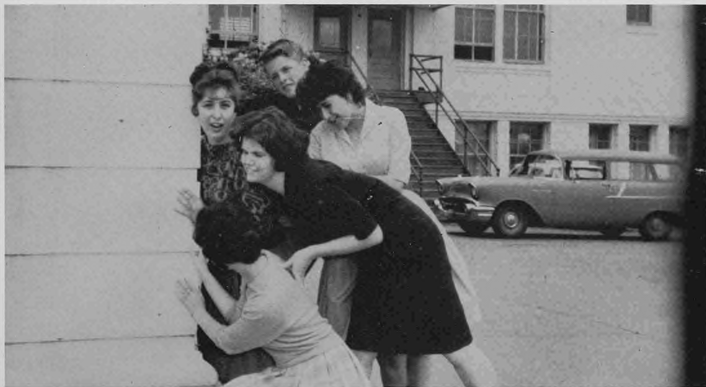
Hey kids! It takes more power than that to move even an old school building like ours. Call on A. C. Johnson & Sons for all types of moving and construction.
