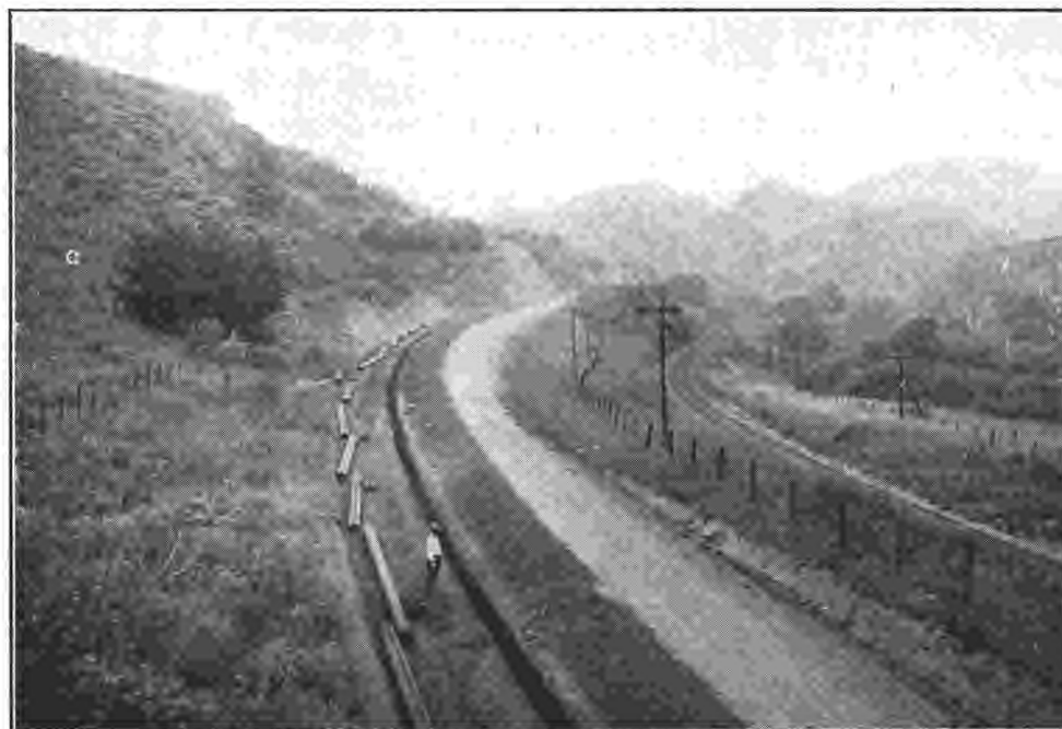
THE MIDWAY GAS CO. PIPE LINE ALONG THE PUBLIC HIGHWAY CARRYING GAS FROM MIDWAY-SUNSET OIL FIELDS TO LOS ANGELES
