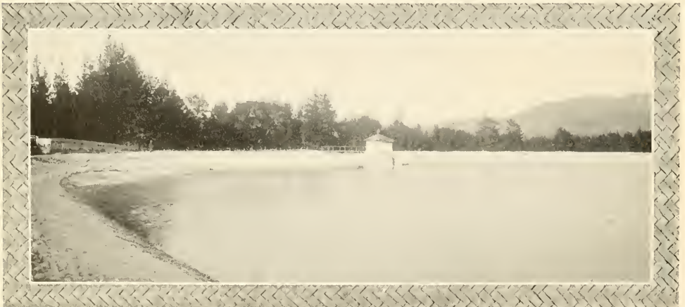
ESPECIAL CARE HAS BEEN TAKEN WITH THE WATER SUPPLY OF THE ENTIRE PENINSULA, AS WILL BE SEEN BY THE PHOTOGRAPH OF THE GREAT RESERVOIR.
