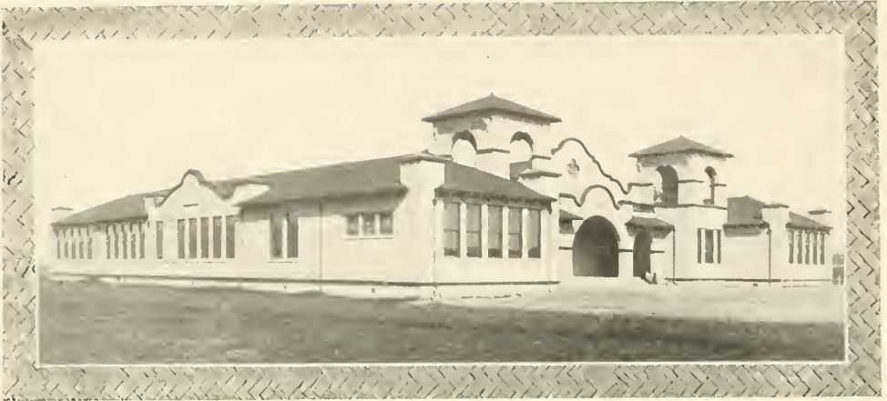
ONE OF THE FINEST HIGH SCHOOLS IN ALL CALIFORNIA IS THE KING CITY SCHOOL, WHICH HAS A LARGE ATTENDANCE. THIS BUILDING COST $35,000 AND IS MODERN IN EVERY DETAIL.
