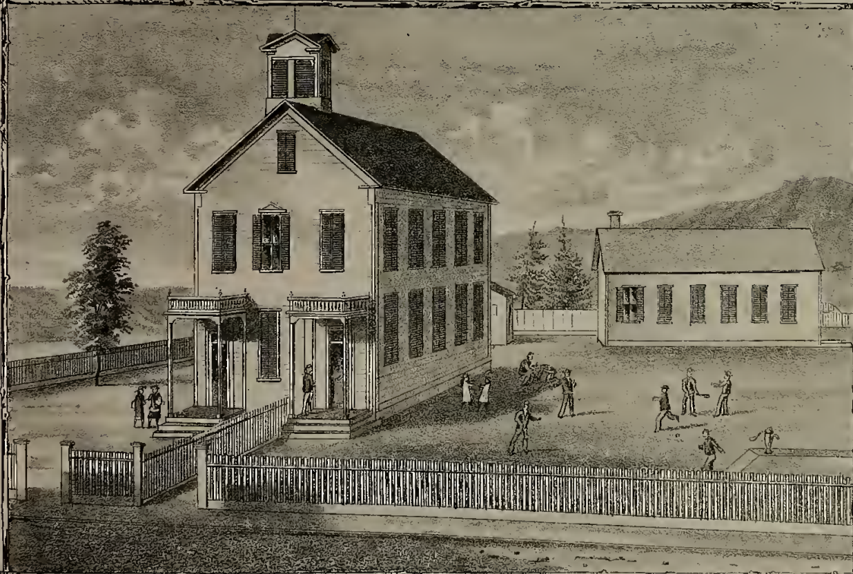
CASTROVILLE SCHOOL BUILDINGS. MONTEREY CO. CAL.
