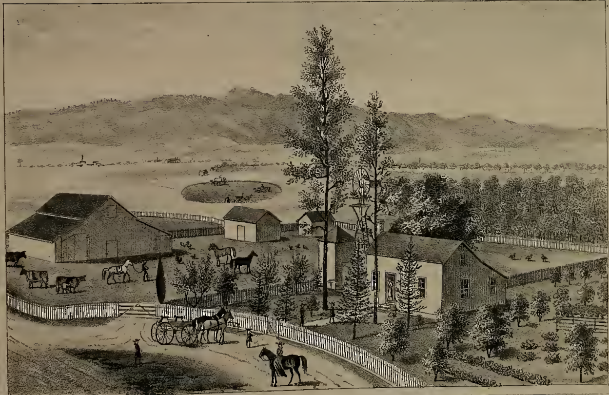
RESIDENCE OF H.W. COTHAN, 3 MILES NORTHEAST OF HOLLISTER, SAN BENITO CO. CAL.
