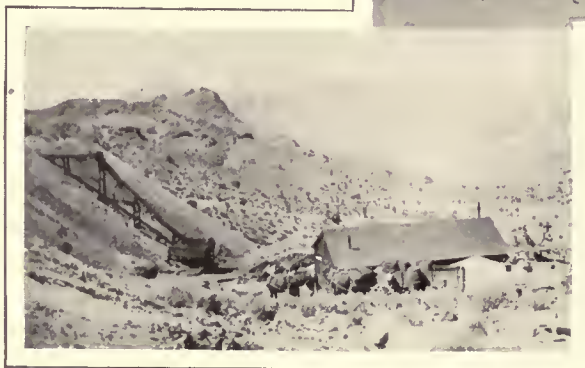
NEVADA-KEYSTONE MINE AND ORE BINS.
