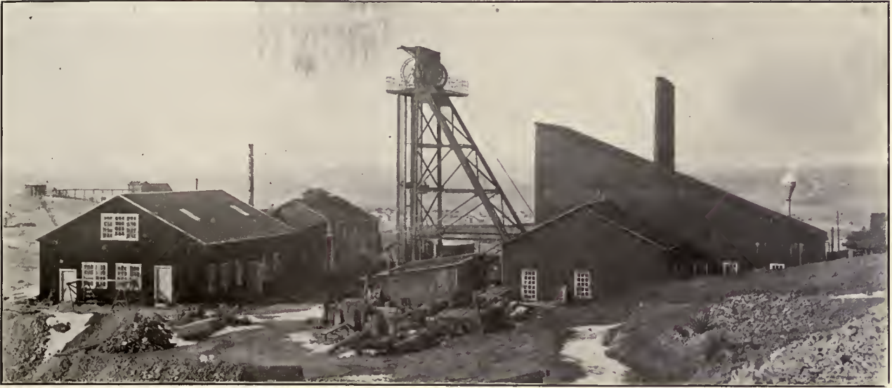
HOISTING PLANT, CONSOLIDATED MINES CO., TOMBSTONE, ARIZONA.
