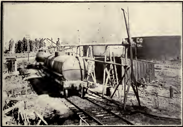
CENTRAL OIL COMPANY'S STORAGE TANKS AT LOS NIETOS, CAL.
