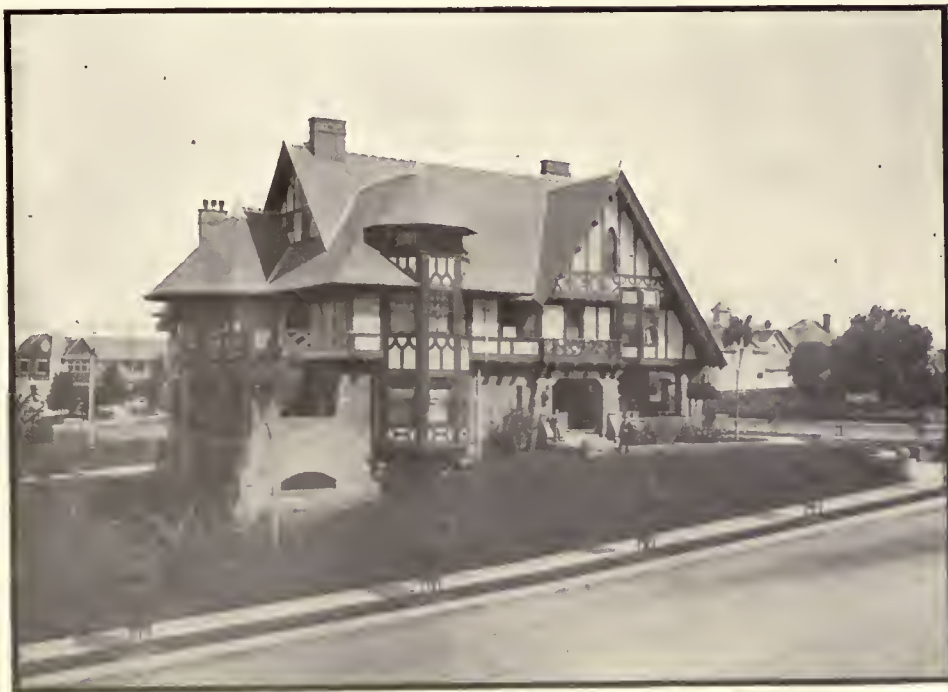
RESIDENCE OF THE LATE JOHN F. FRANCIS.
