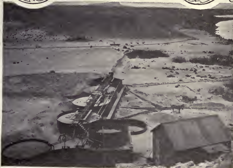
CYANIDE TANKS AT MILL
