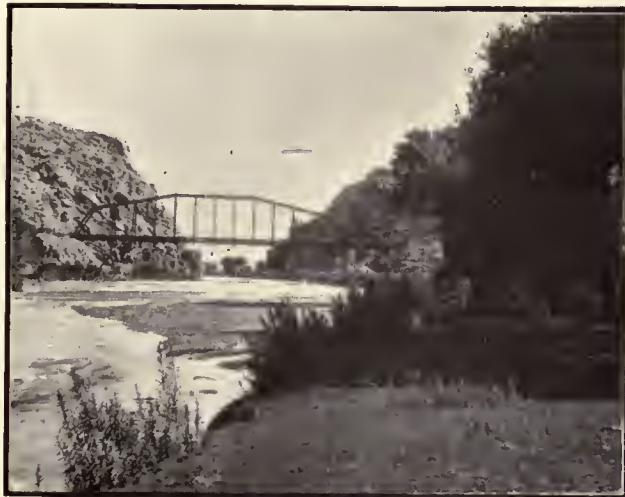
SANTA FE BRIDGE OVER THE MOJAVE RIVER.
