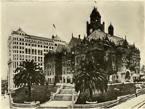
THE LAWS' DIGNITY OF TODAY Present Court House and Hall of Records
