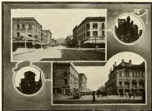
BUILDING NOW COVERING OLD PASADENA
