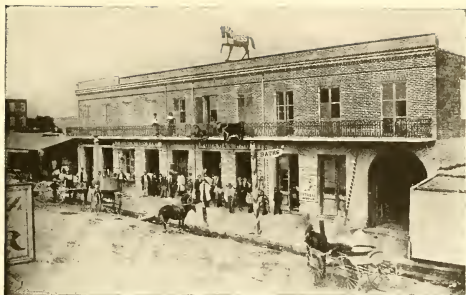
MAIN AND TEMPLE STREETS, OPPOSITE PRESENT POST OFFICE
