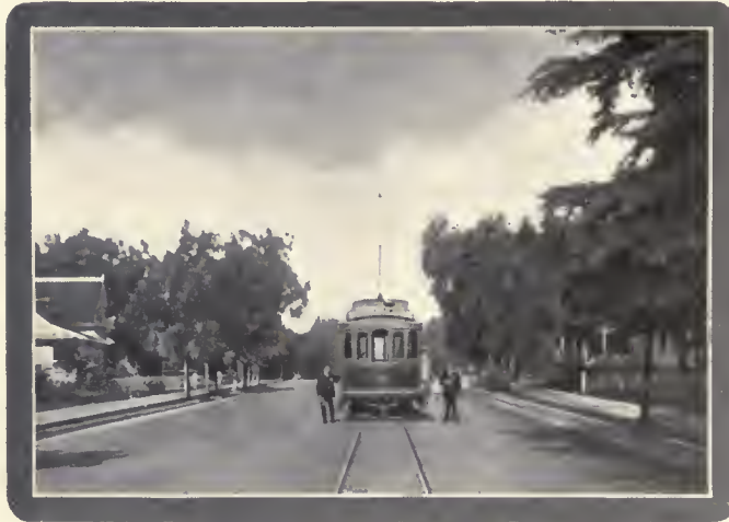
NORTH THIRD STREET.
