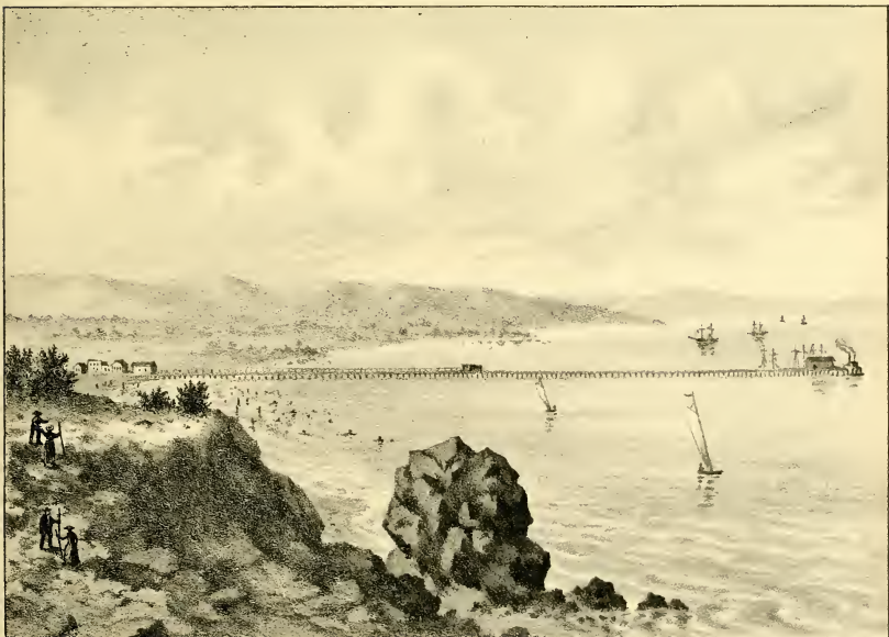
VIEW OF WHARF AT SANTA BARBARA, CAL. J. P. STEARNS, PROP'R.
