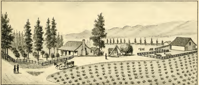
RESIDENCE & RANCH OF SAMUEL CONNER, SANTA MARIA, SANTA BARBARA CO. CAL.
