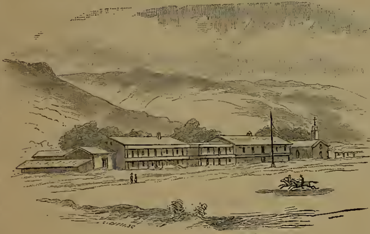
MISSION CHURCH AND BUILDINGS AT SONOMA.
