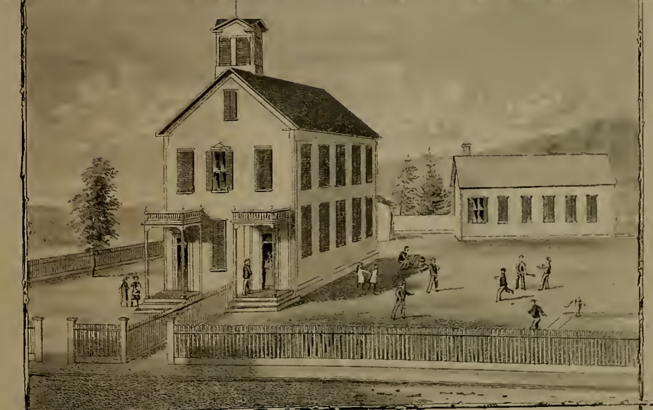
CASTROVILLE SCHOOL BUILDINGS. MONTEREY CO. CAL.
