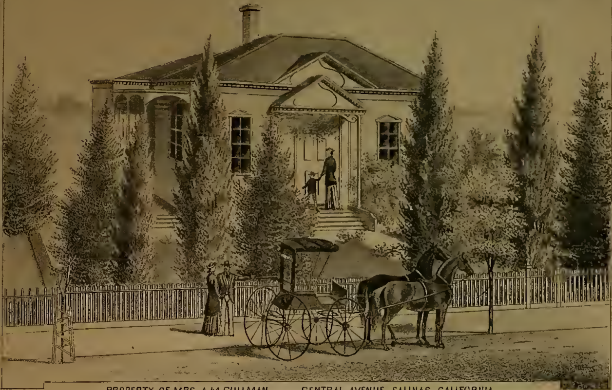
PROPERTY OF MRS A.M.CULLMAN. CENTRAL AVENUE SALINAS CALIFORNIA,
