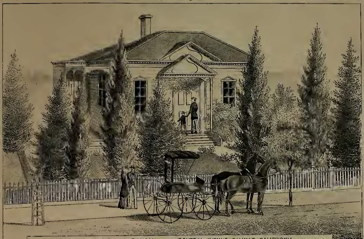
PROPERTY OF MRS A.M.CULLMAN. CENTRAL AVENUE SALINAS CALIFORNIA.
