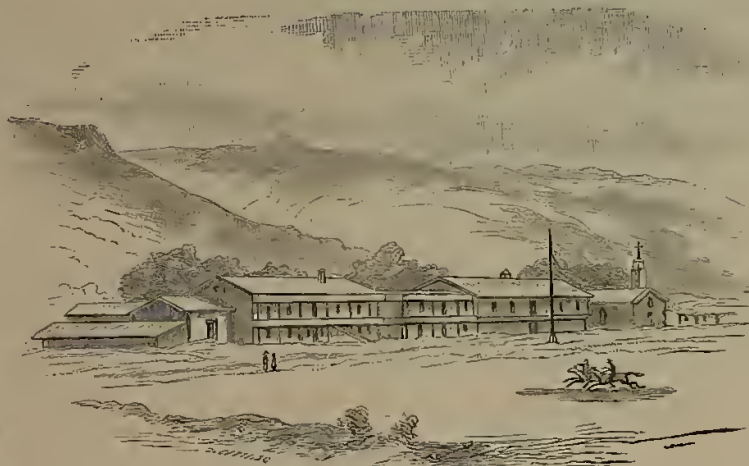
MISSION CHURCH AND BUILDINGS AT SONOMA.
