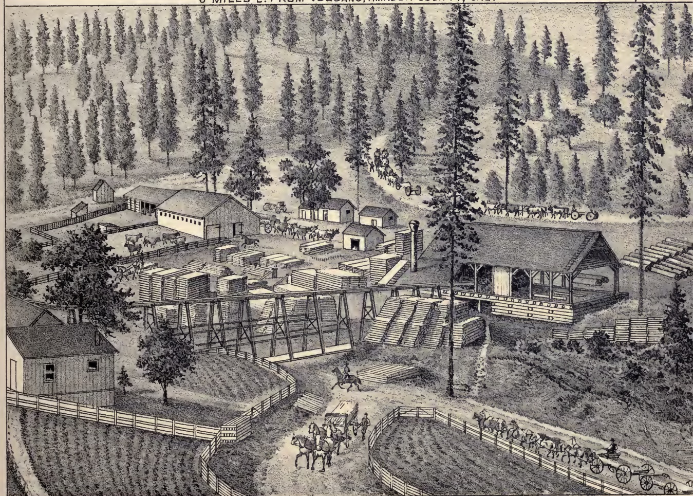
RESIDENCE AND SAWMILL OF F. M. WHITMORE, ANTELOPE CREEK, NEAR VOLCANO, AMADOR COUNTY, CAL.
